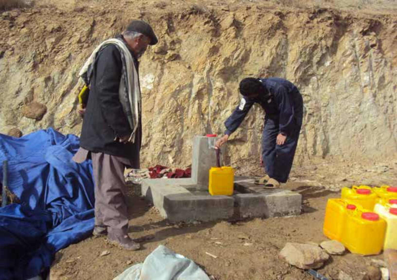
Water Supply Project in Kabul Financially Supported by NCA-2022
