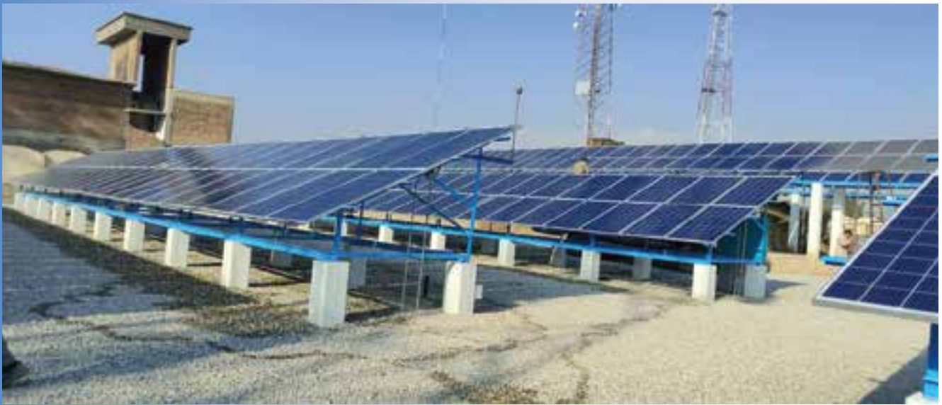
Fig.9 - Solar system and Water supply project in Laghman province, financially supported by UNICEF, 2022.
