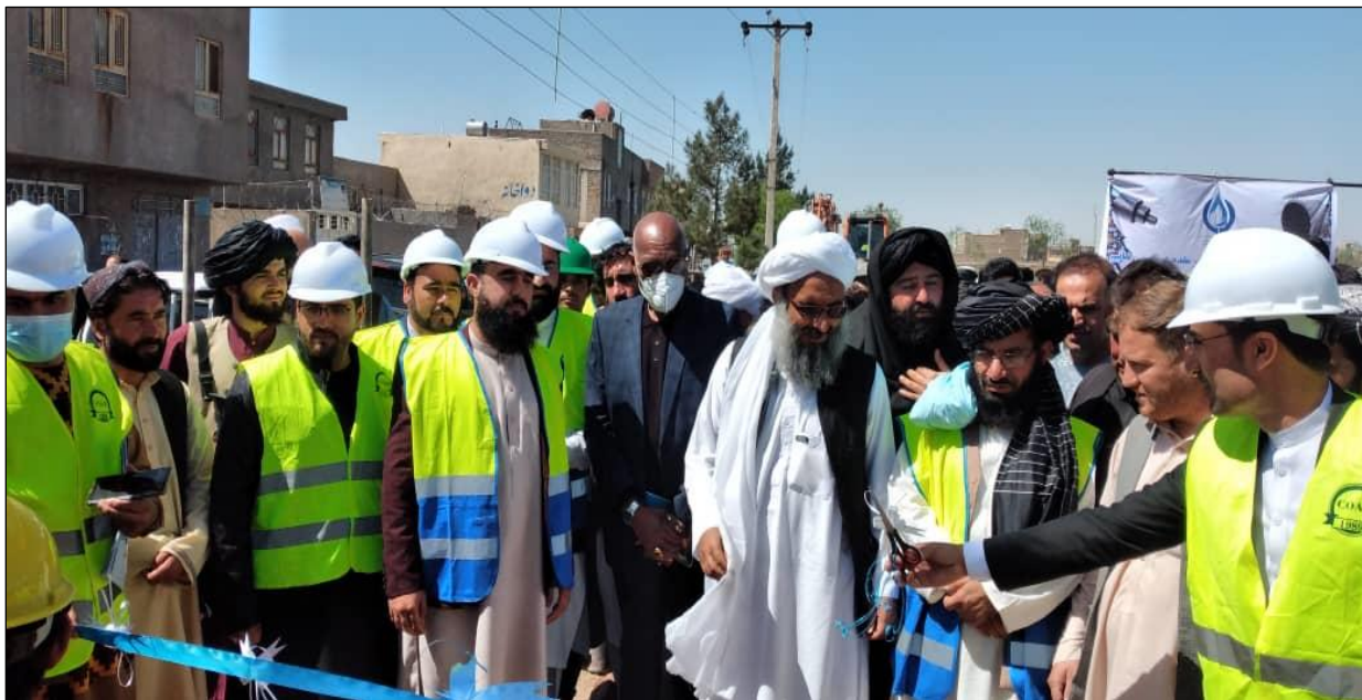
Inauguration of Herat urban water supply pipe scheme extension project in the presence of high authorities of government, UNICEF, COAR and community elders.
